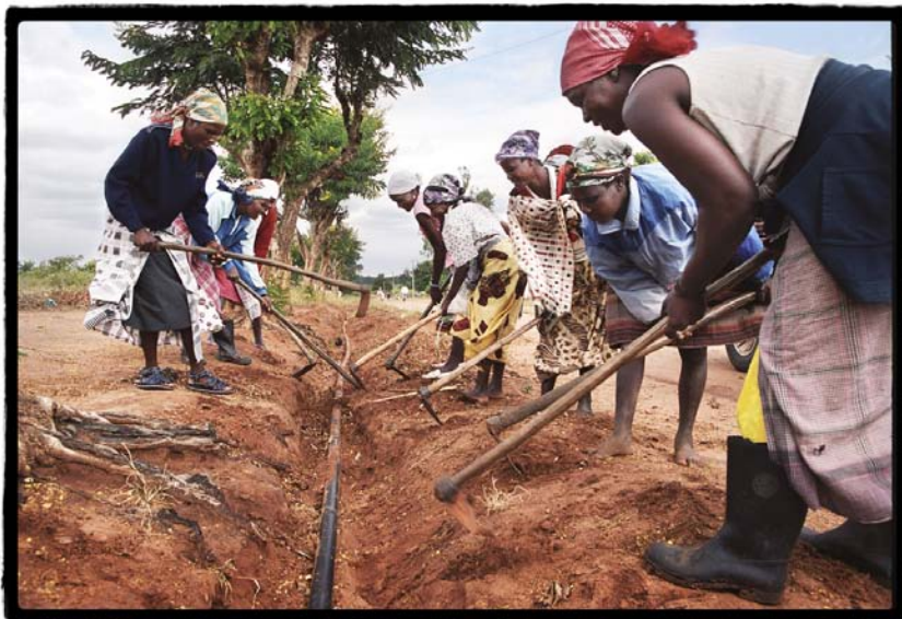
The public are an enormous help: digging a pipeline in Mozambique.
